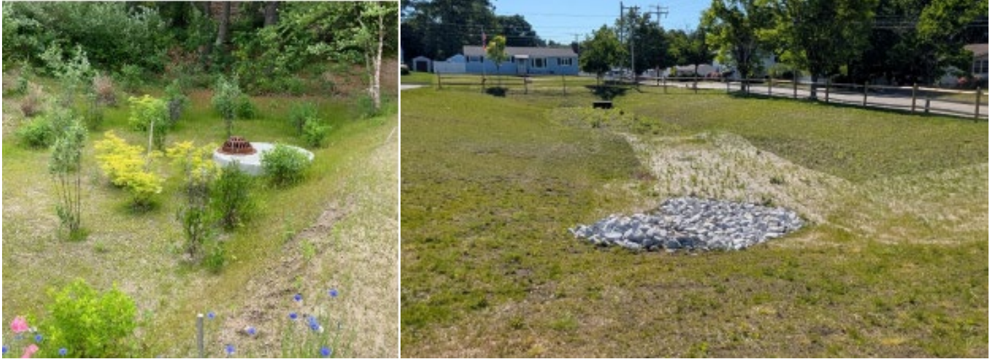
Figures 3-4: Two bioretention basins constructed for stormwater runoff treatment in Manchester, NH (source: Comprehensive Environmental Inc.)
