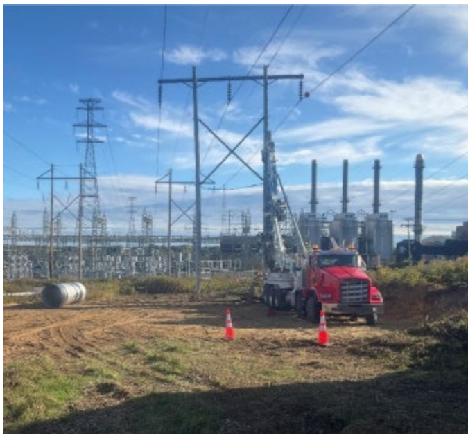
Figure 3: Transmission structure replacement.
