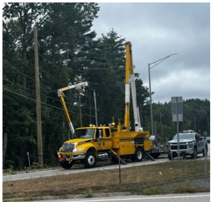
Figure 4: Photo of distribution pole replacement.
