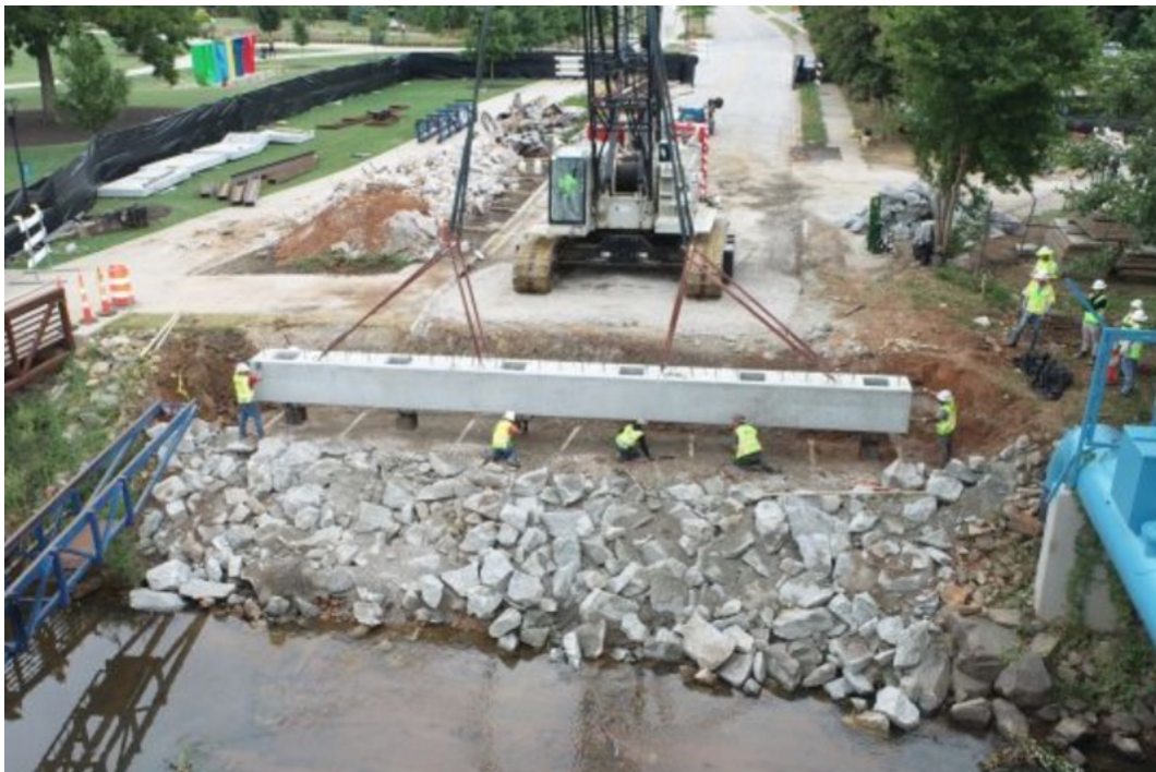
FIGURE 7: ACCELERATED BRIDGE CONSTRUCTION IN GREENVILLE, SC
