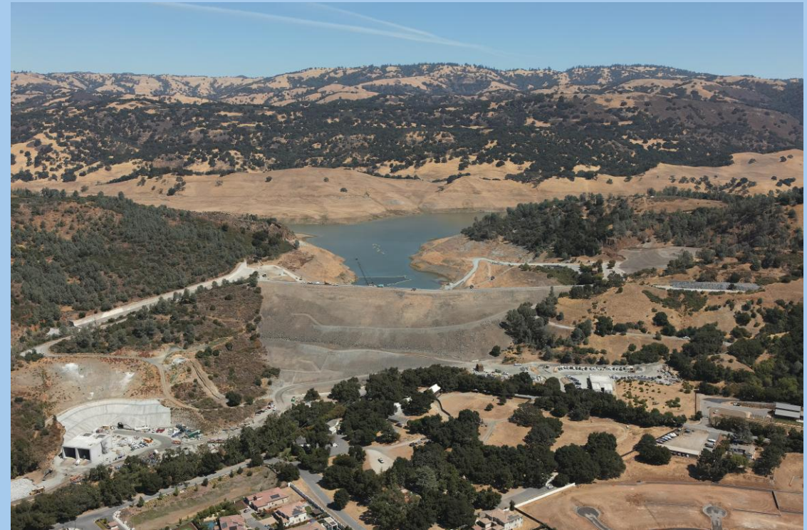
Anderson Dam, Santa Clara Valley Water District, California
