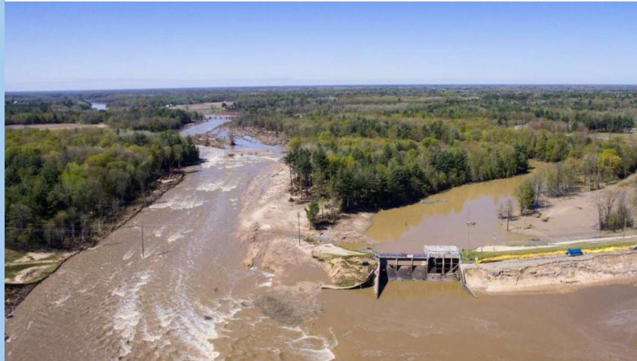
Edenville Dam – Post Failure
