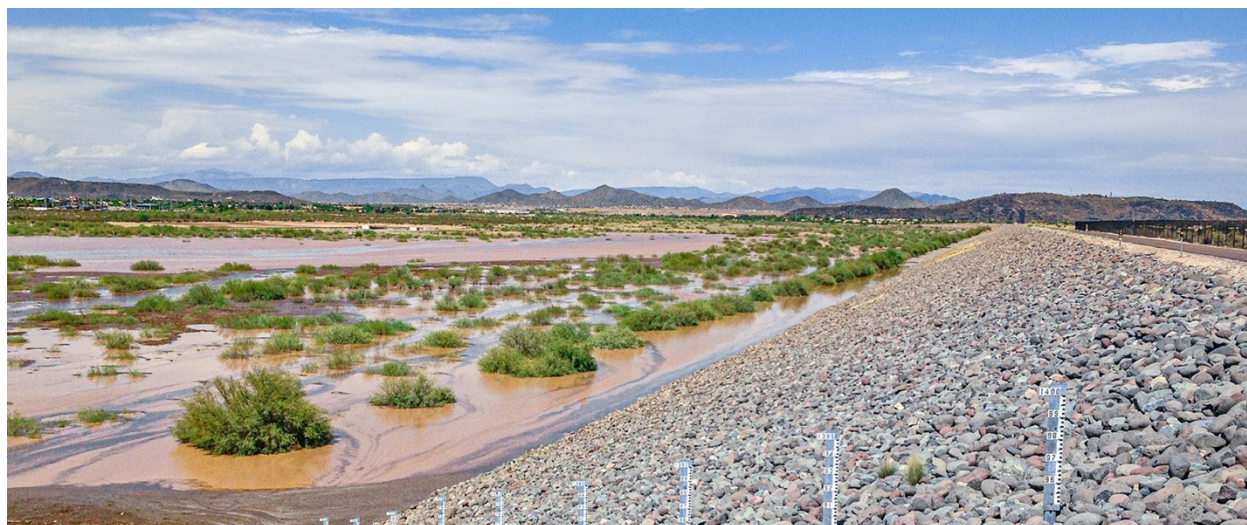
Figure 2 – Levee in Maricopa County, Arizona Flood Control District of Maricopa County
