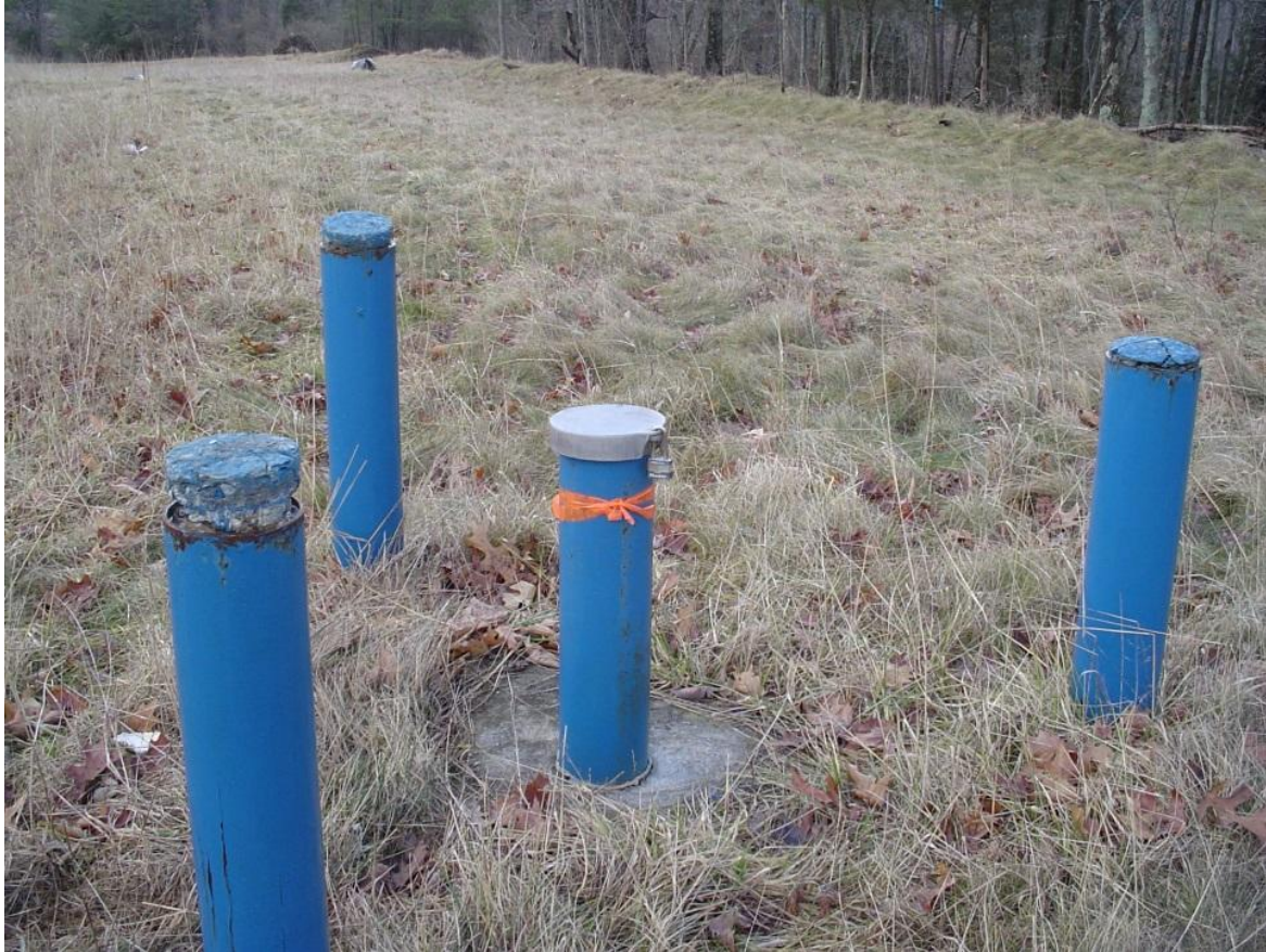
Groundwater monitoring well
