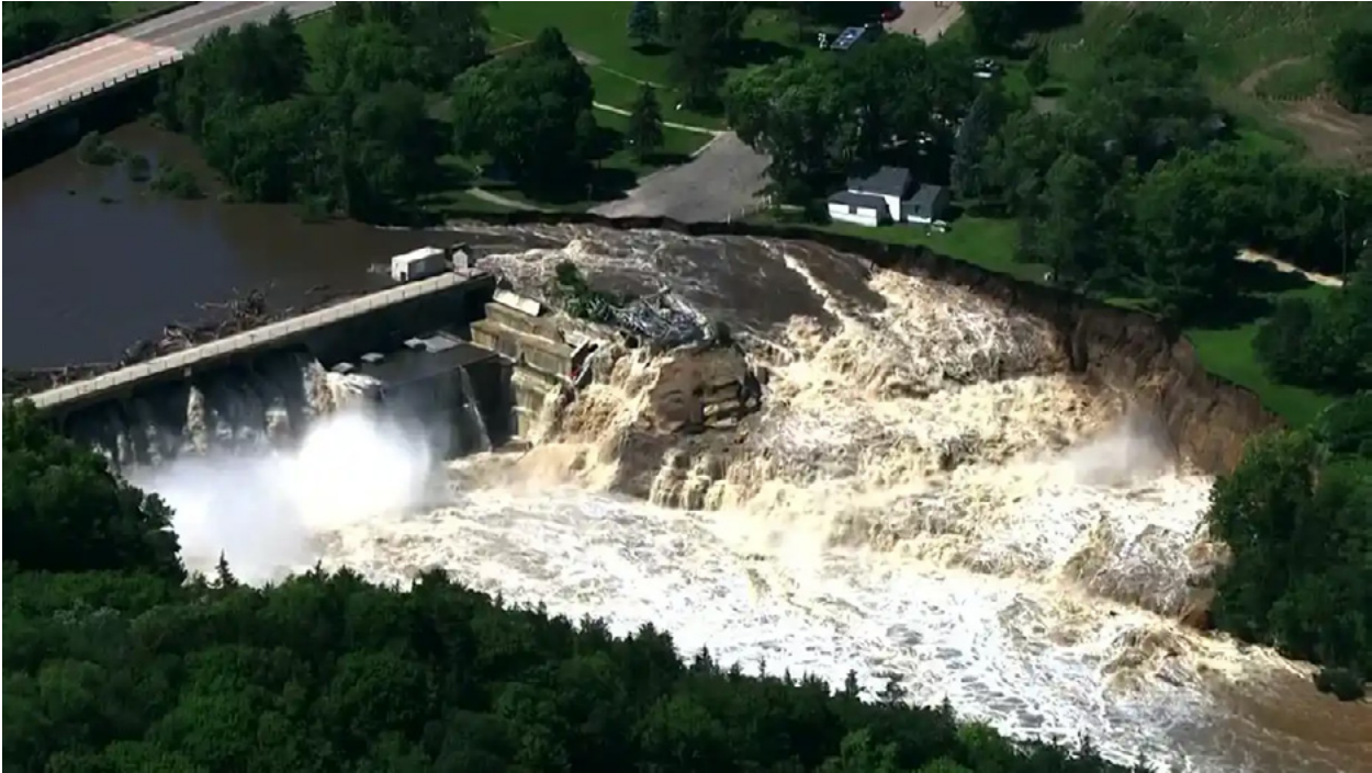
FIGURE 5: FAILURE OF THE RAPIDAN DAM IN SOUTHERN MINNESOTA
