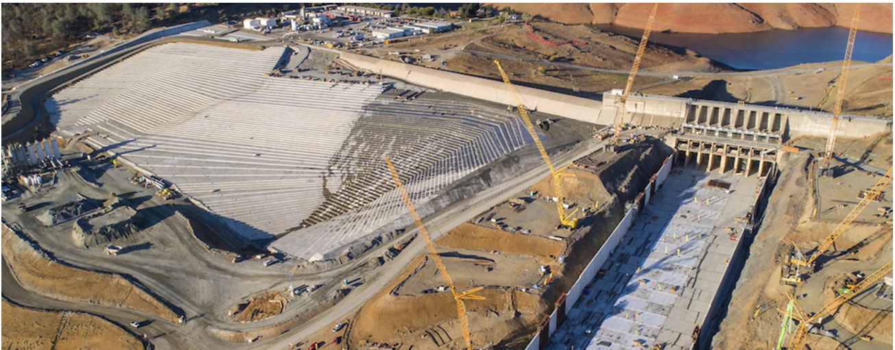
Photo 5: The Oroville Dam Main Spillway and Emergency Spillway Repair. (Photo Credit: Department of Water Resources)
