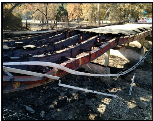
The Mulholland Highway Bridge over Triunfo Creek near Malibu Lake was severely damaged by the Woolsey Fire in 2018 (Left). It was reconstructed in 2020 (Right).
