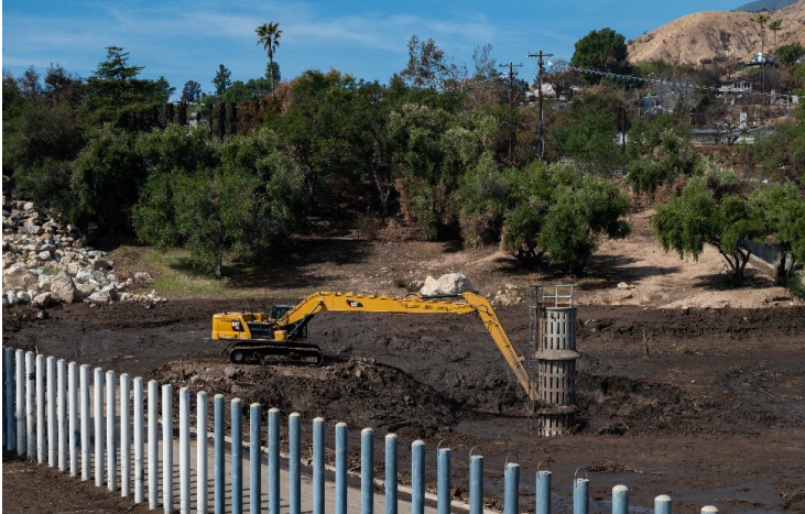
Photo 2: Rubio Canyon Debris Basin Dam – Post-Eaton Fire Sedimentation (Photo Credit: Los Angeles County Public Works)
