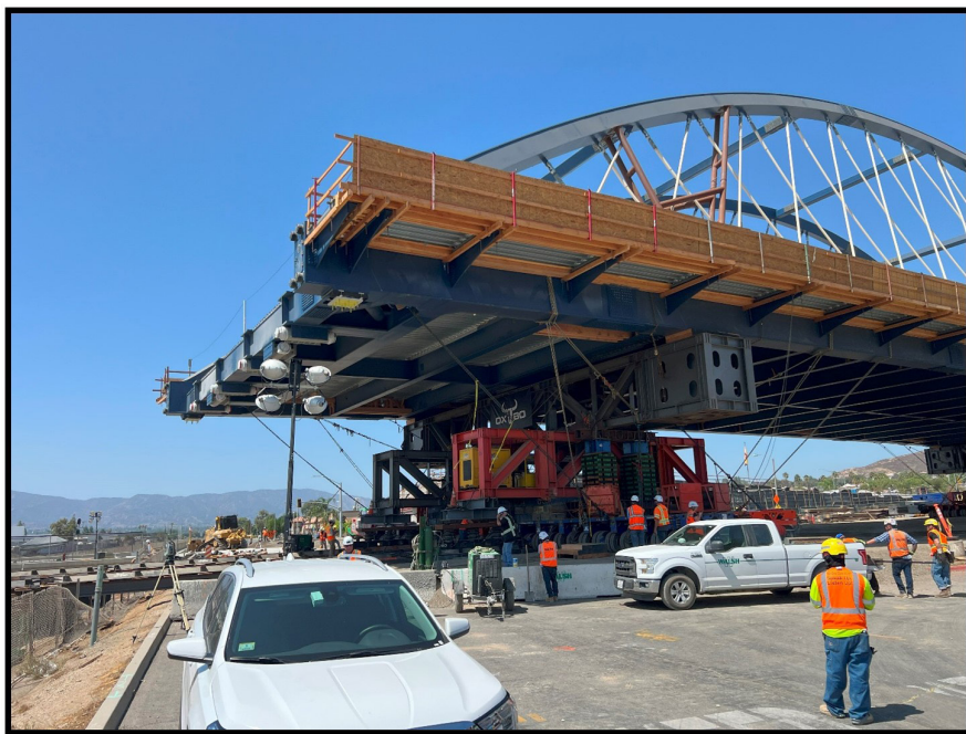
Self-propelled modular transporters, a form of Accelerated Bridge Construction, are used to move a bridge from a staging area to its final location (Source: Biggs Cardosa Associates).
