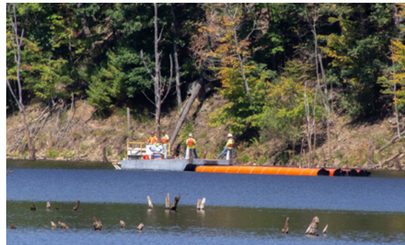
Figure 6: Boom installation at North Bend State Park Dam
