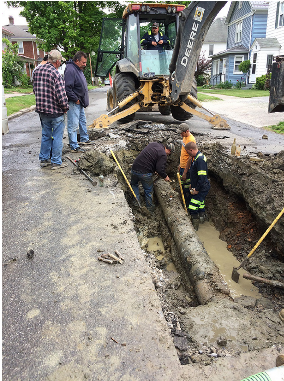
Figure 6: Water line repairs
