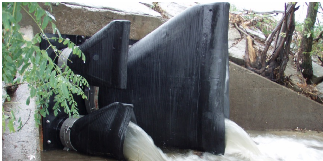
Figure 11: Duckbill check-valves in Huntington, WV
