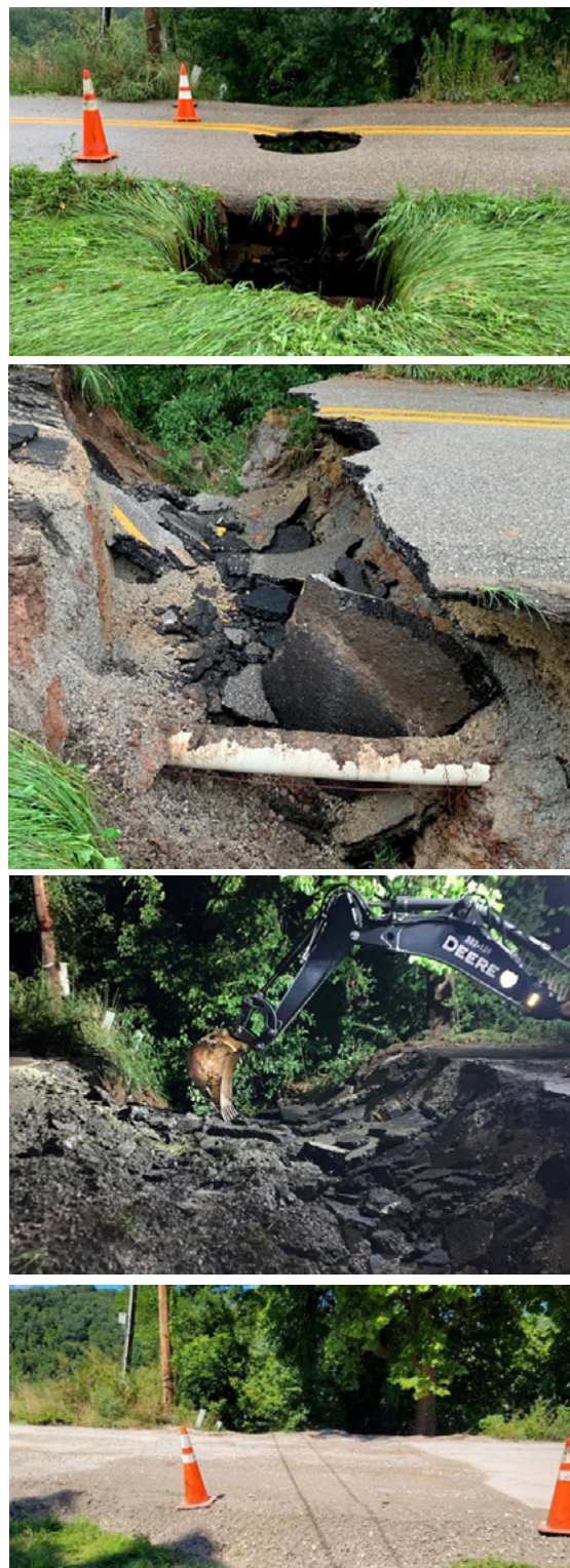
Figure 9: Sissonville, WV sinkhole under the road. The WVDOH was able to repair and reopen the road in just over 6 hours.
