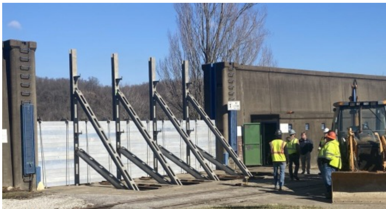
Figure 4: Floodwall Erection in Huntington, WV
