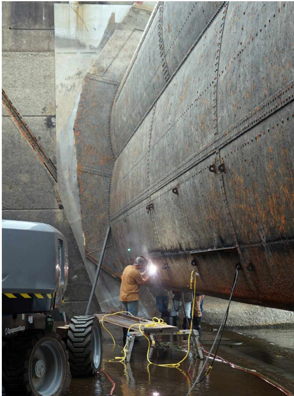
Figure 2: USACE Roller Gate Repairs
