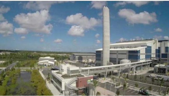
The Palm Beach Renewable Energy Facility 2, completed in 2015, is the newest municipal waste-to-energy facility in the country. It cost $672 million and can process up to 3,000 tons of municipal solid waste per day.
