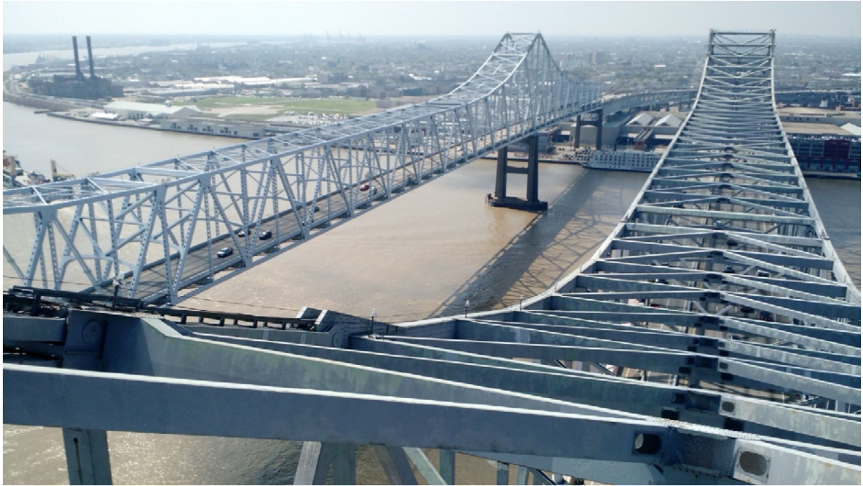
Figure 1: Two of Louisiana's many Major River Crossings – Crescent City Connections 1 and 2, in New Orleans, Louisiana.
