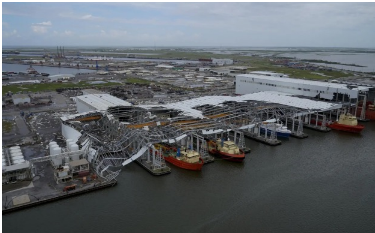
Figure 3: Hurricane Ida Damage at Port Fourchon
