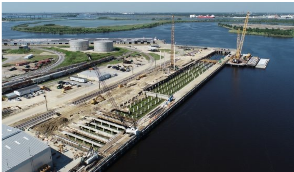
Figure 4: CMAR Berth Rehabilitation at Port of Lake Charles
