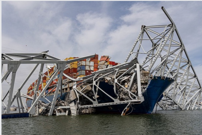
Figure 4. Wreckage from the Francis Scott Key Bridge collapse Source: USACE
