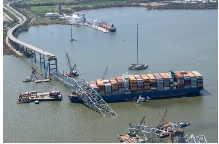
Figure 3. Francis Scott Key Bridge after its collapse in March 2024
