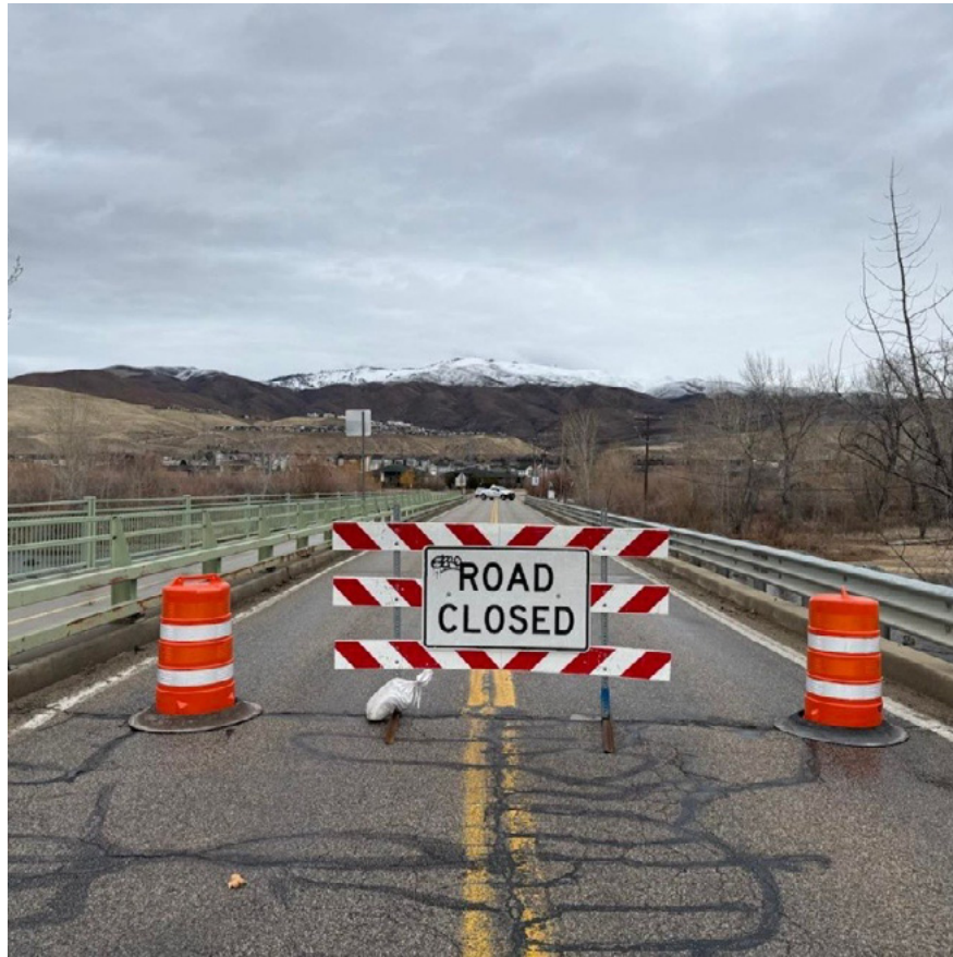
Figure 6. Eckert Road Bridge Closure
