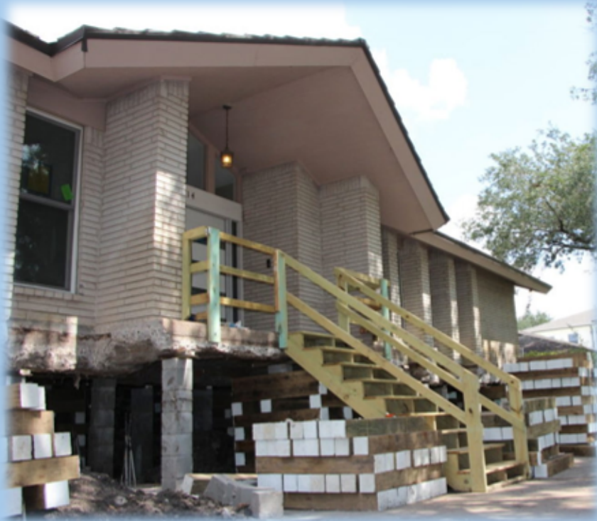
ELEVATION Raising existing structures
