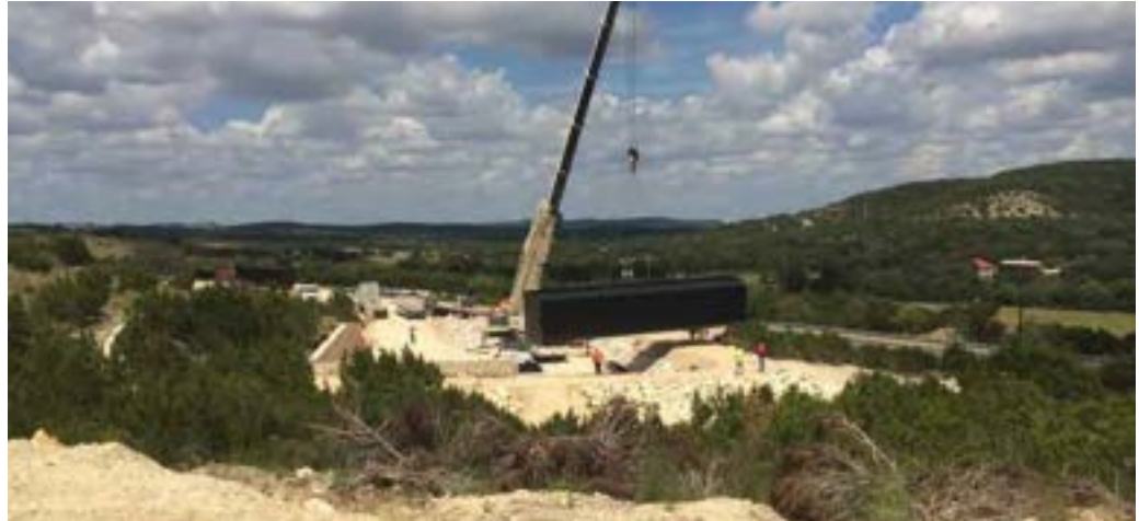
FIGURE 9. Installation of Packaged 110,000 GPD Wastewater Treatment Plant in Kendall County
