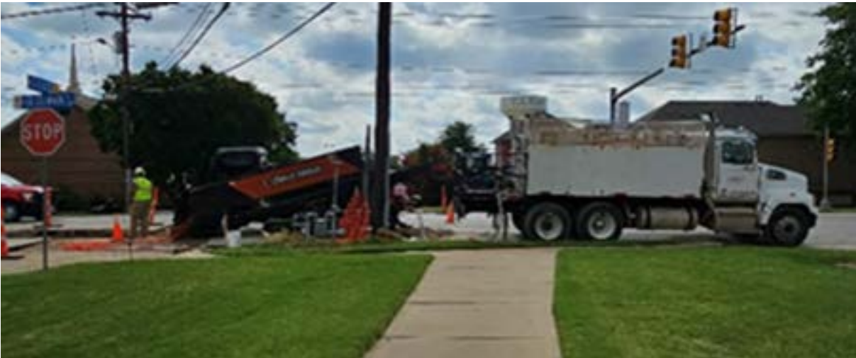
FIGURE 1. Replacing existing pipe through Pipe Bursting Methods in Euless, TX
