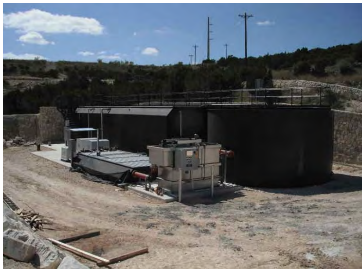
FIGURE 10. Completed Installation of above Packaged WWTP in Kendall County, TX
