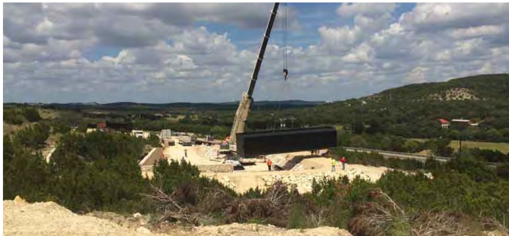
FIGURE 9. Installation of Packaged 110,000 GPD Wastewater Treatment Plant in Kendall County
