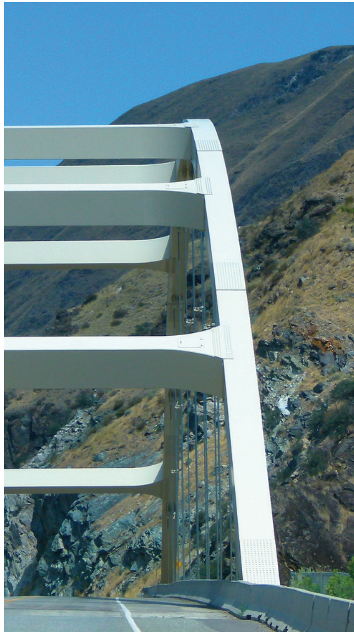
Time Zone Bridge located in Riggins, Idaho. This tied arch bridge spans the Salmon River and provides a critical north-south connection.
