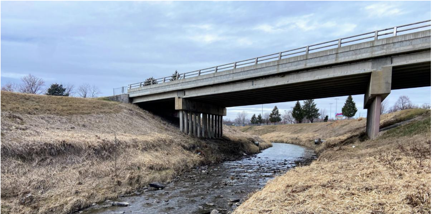
FIGURE 3. TYPICAL BRIDGE IN GOOD CONDITION
