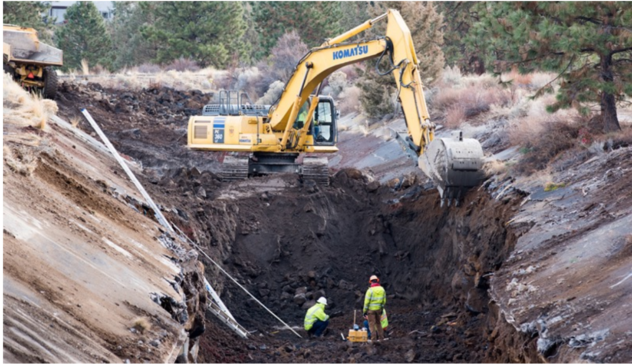
Canal piping project. Source: Central Oregon Irrigation District
