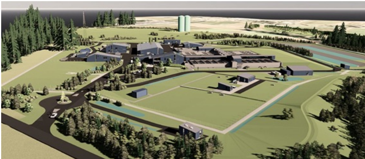
Source: Portland.gov - About the Bull Run Filtration Project
