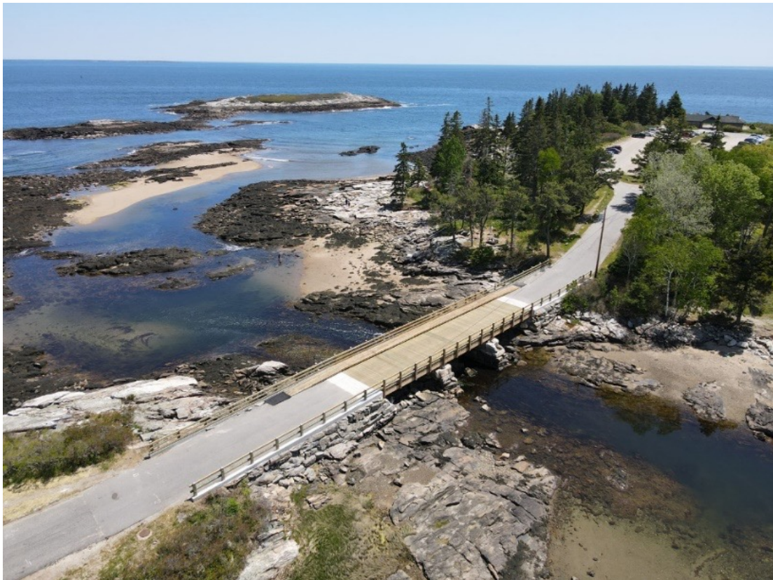
FIGURE 2. NEW BRIDGE CONSTRUCTION TO GIFFITH'S HEAD IN REID STATE PARK XI
