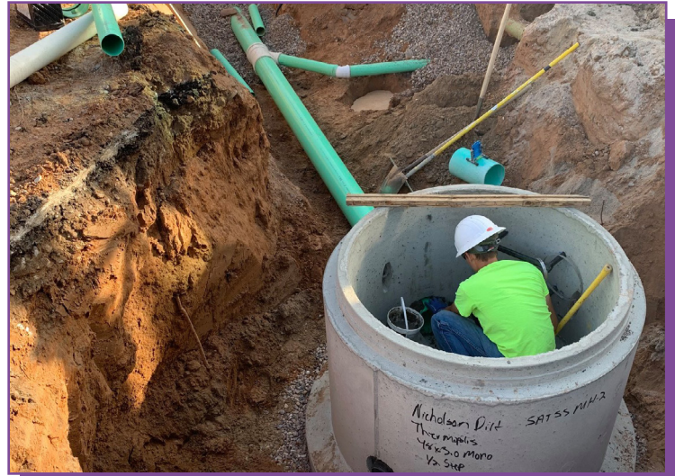
SPRINGVIEW STREET SEWER REPLACEMENT, THERMOPHIS, WY
