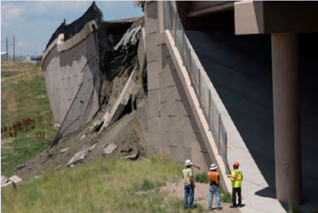
FIGURE 1: COLLAPSE OF US-36 (SOURCE: CPRNEWS)
