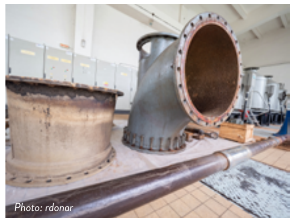
AXIAL HYDRODYNAMIC FLOW PUMP IN WASTEWATER PLANT.
