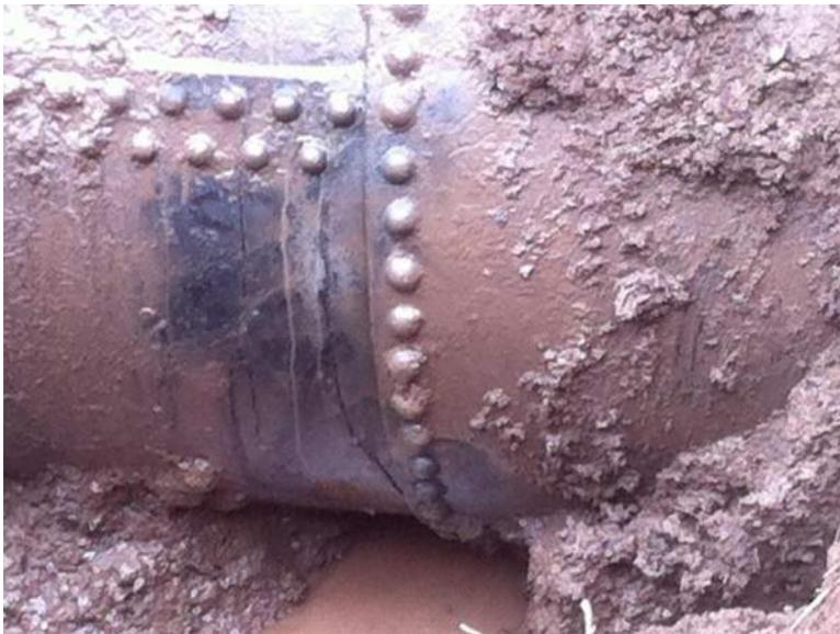
The condition of the drinking water infrastructure in the City of Duluth is poor. The City has 433 miles of piping. Durable cast-iron pipe, as shown in the above photo, was installed in the 1880s and 1890s and can last for 120 to 130 years, meaning it is now coming to the end of its design service life. The piping installed from 1910 to 1920, projected to last about 100 years, is also due to be replaced. Pipe installed in the 1960s and 1970s, which has had a life span of 50 to 60
