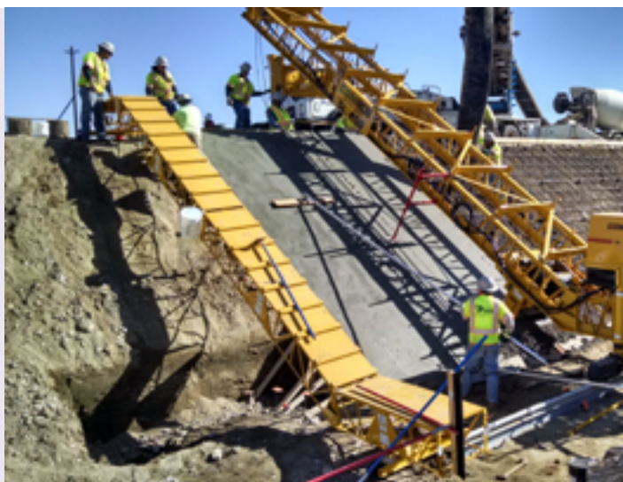
LEVEE CONSTRUCTION IN PUEBLO, COLORADO
