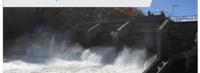
Iowa Falls Hydroelectric Dam, 2016
