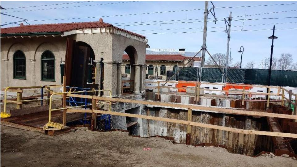
*Excavation to install lift required to comply with ADA regulations at Westerly Station – Spring 2020*
