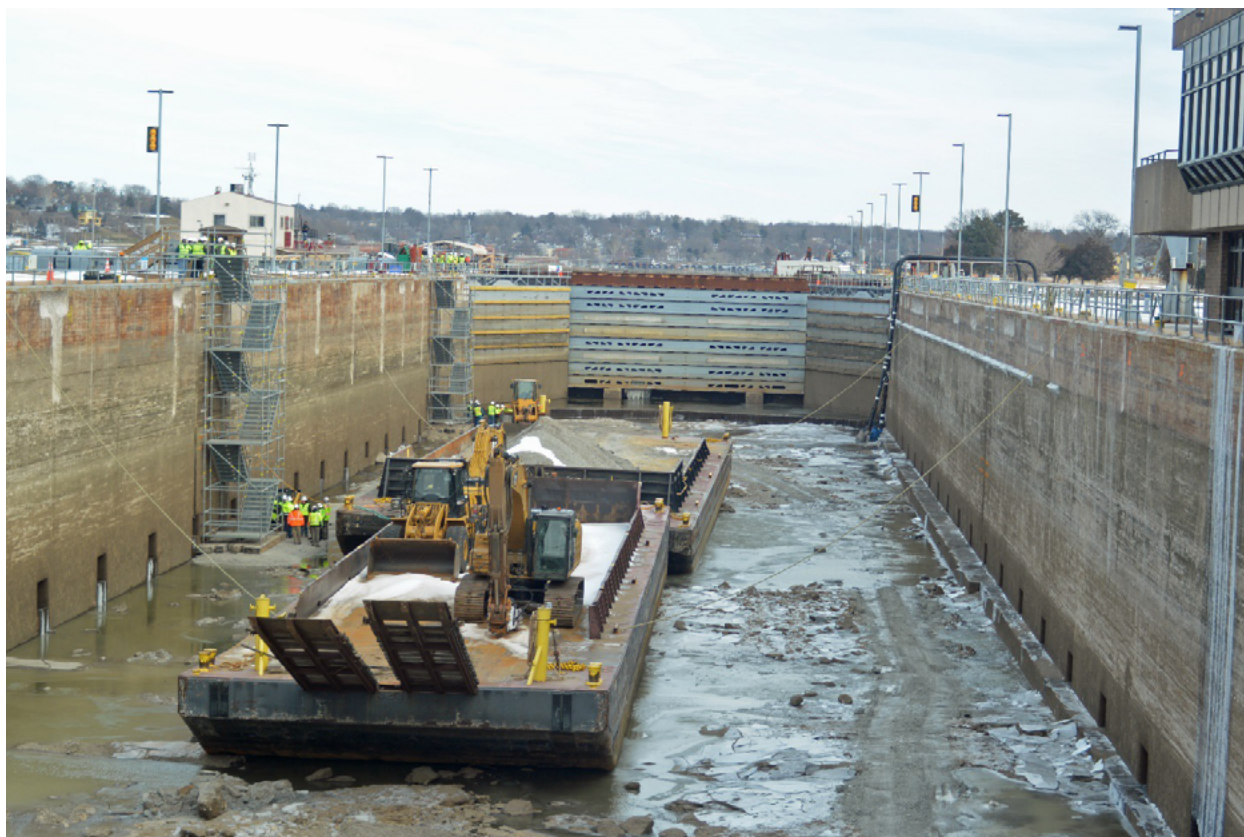
FIGURE 4: MISSISSIPPI LOCK AND DAM NO. 15 JANUARY 2022 DEWATERING
