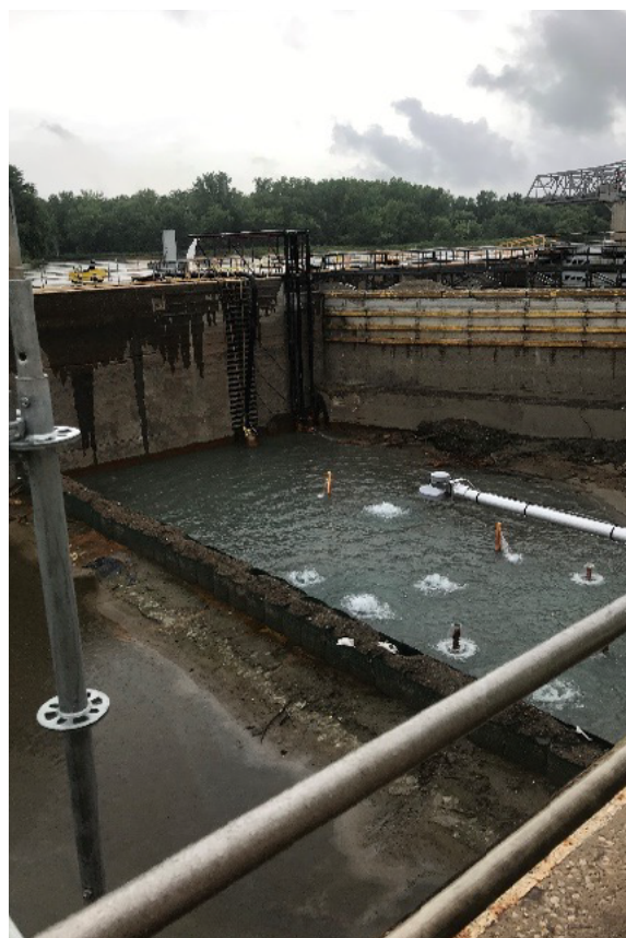
FIGURE 7: PEORIA LOCK AND DAM DEWATERING, JULY 2020
