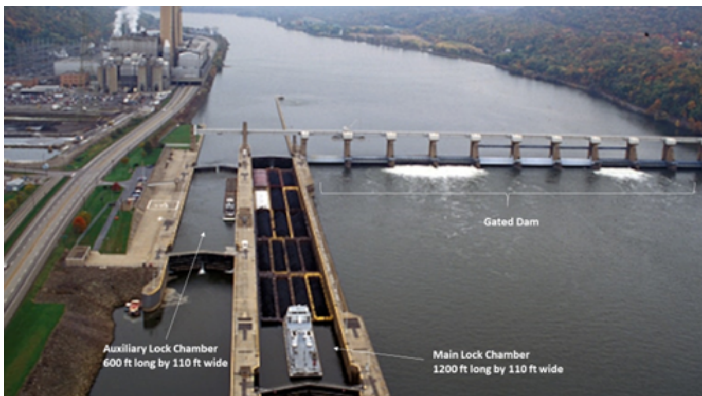
FIGURE 4. TYPICAL CONFIGURATION OF OHIO RIVER NAVIGATION LOCKS AND DAMS
