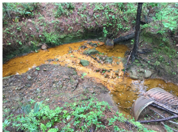
Deteriorating and collapsed stormwater infrastructure conveying polluted water. (Photo courtesy of Barry Fagan.)
