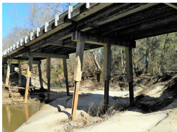
Scoured bridge piers in Barbour County, Alabama. (Photo provided by ALDOT.)
