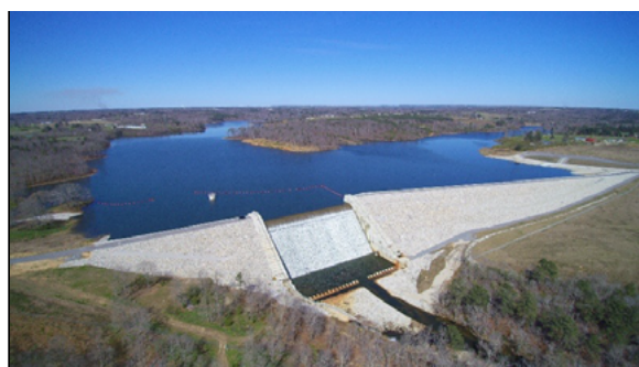
Recently completed water supply clay core/rockfill embankment dam with a concrete spillway.
